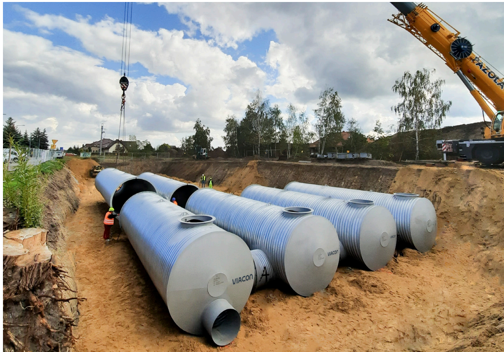
D3300 mm, L-10.00 m, V-86 m 3 , 2 pcs. and D3000 mm, L-5.20 m, V-37 m 3 , 1 pc.
